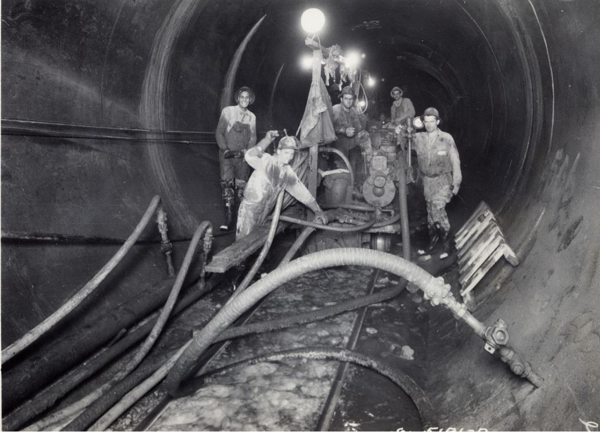
Workers in the Rondout-West Branch Tunnel
